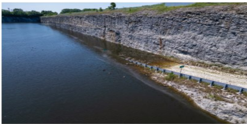
A ramp leading into the Deep Tunnel water reservoir north of the Thornton Quarry is partially submerged Monday following a rainy June and early July. STACEY WESCOTT/CHICAGO TRIBUNE
